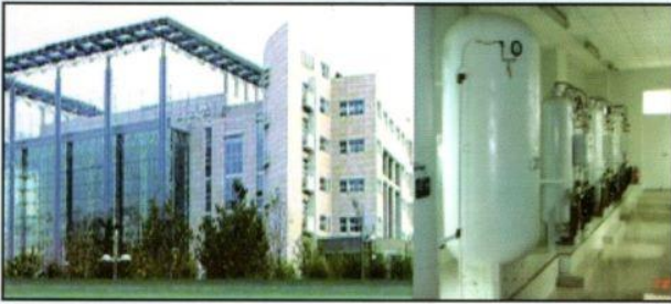
The First Affiliated Hospital of Jilin University, China A 1200 Bedded Hospital having equivalent 375 D Type oxygen Cylinder capacity - AS-L Triplex system running since 2005
