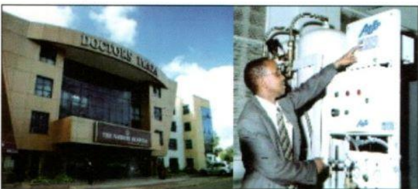
The Nairobi Hospital, Kenya A 350 Bedded Hospital having equivalent 125 D Type oxygen Cylinder capacity - AS-L system running since 2005
